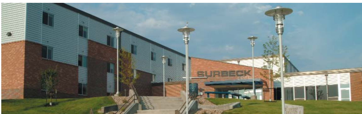
Howard Peterson Hall was completed in the summer of 2004. It was constructed adjacent to the south end of the Surbeck Center.
